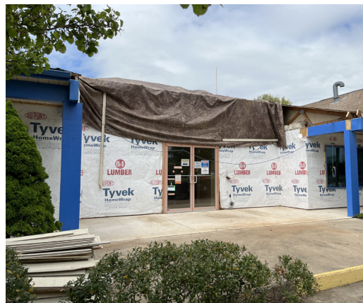
Framing for front vestibule
